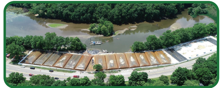
Aerial view of sediment dewatering operation
