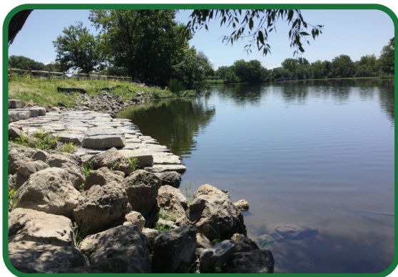
Erosion bank stabilization with pedestrian access
