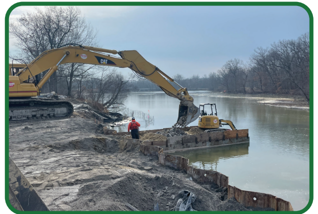
Loading of stone for fish substrate placement
